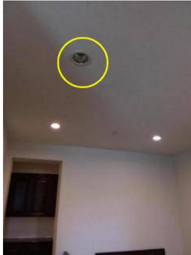
Photo 19-2 2nd floor stairwell
