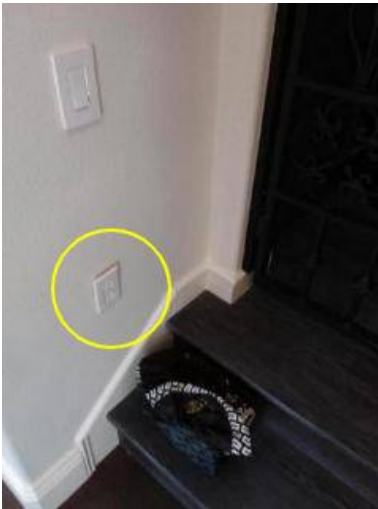
Photo 13-1 Near the wine storage room
