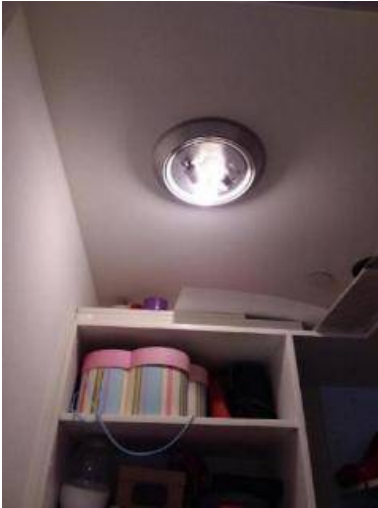
Photo 14-1 Front right corner bedroom closet
